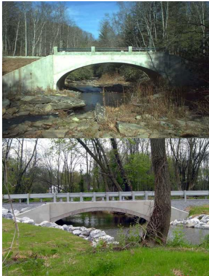
Figure 5.3. Examples of Bottomless Arched Culvert Crossings
