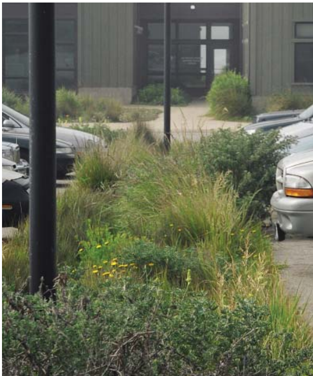
Example of Bioswale in Parking Lot (UCSC Seymour Marine Discovery Center) ( Figure 33)
