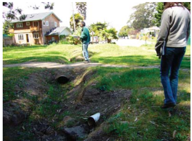
Existing Drainage Channel (Figure 70)
