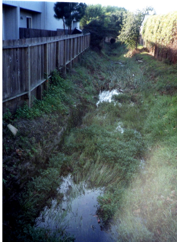
Figure 3.10. Moran Creek—Open Channel with Urban Encroachment
