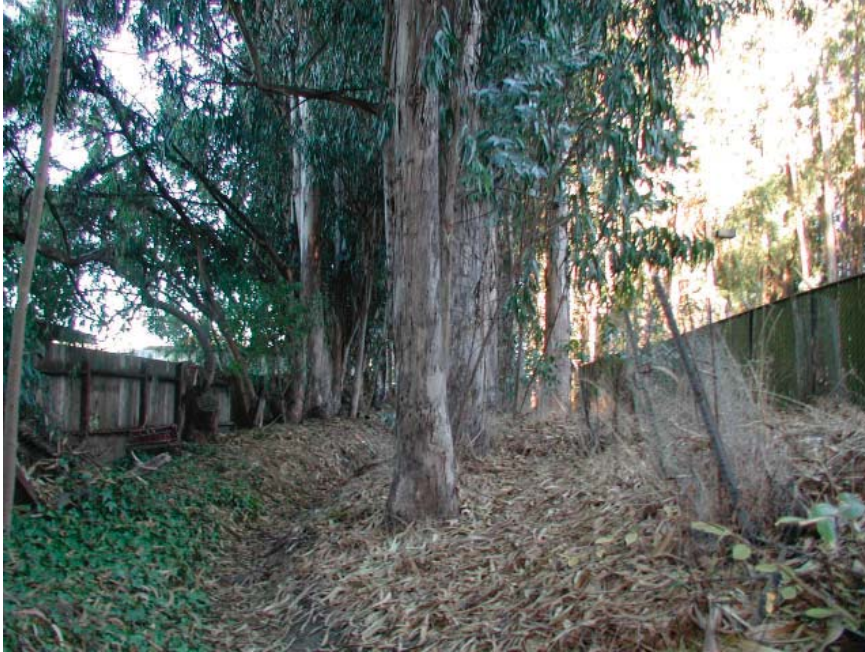
Existing Conditions at Critical Windbreak (Before) (Figure 74)
