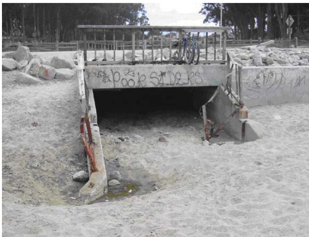
Box Culvert at Moran Lake Beach (Photo: FCE) (Figure 20)
