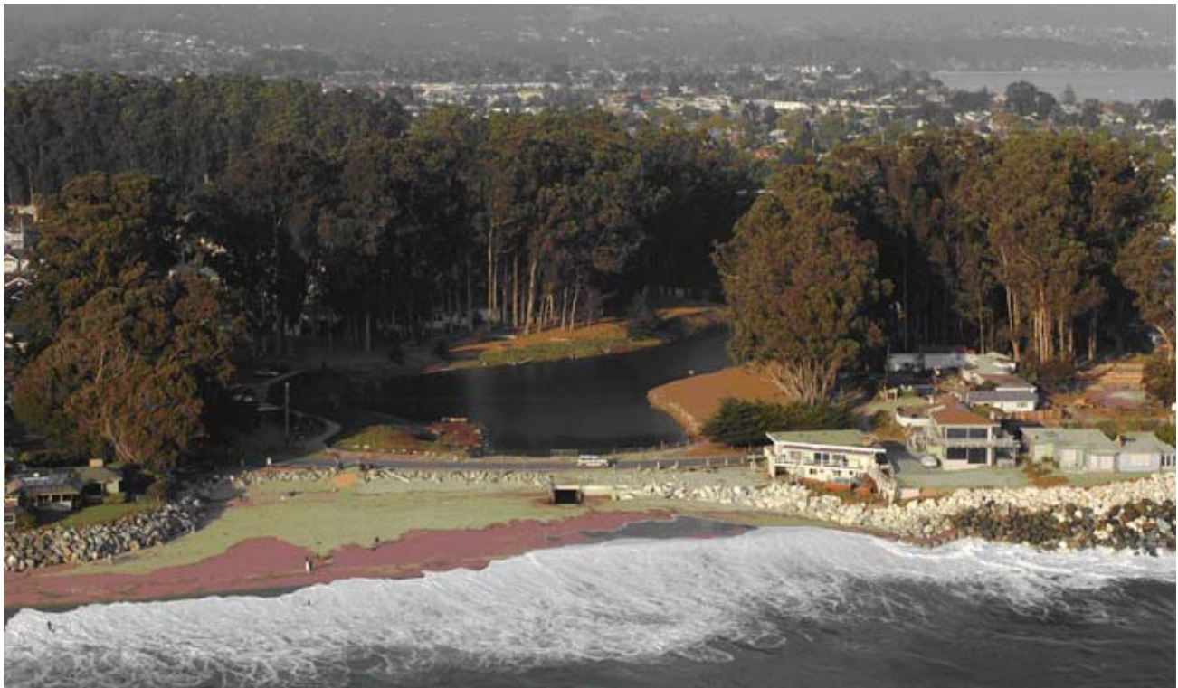
Moran Lake Outlet (September 2002) Photo: California Coastal Commission (Figure 19)
