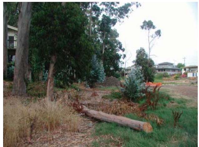
Saturated Area Causing Tree Failure (Figure 24)
