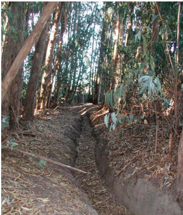
Existing Drainage Channel at D. A. Porath Sanitation Facility (Figure 23)
