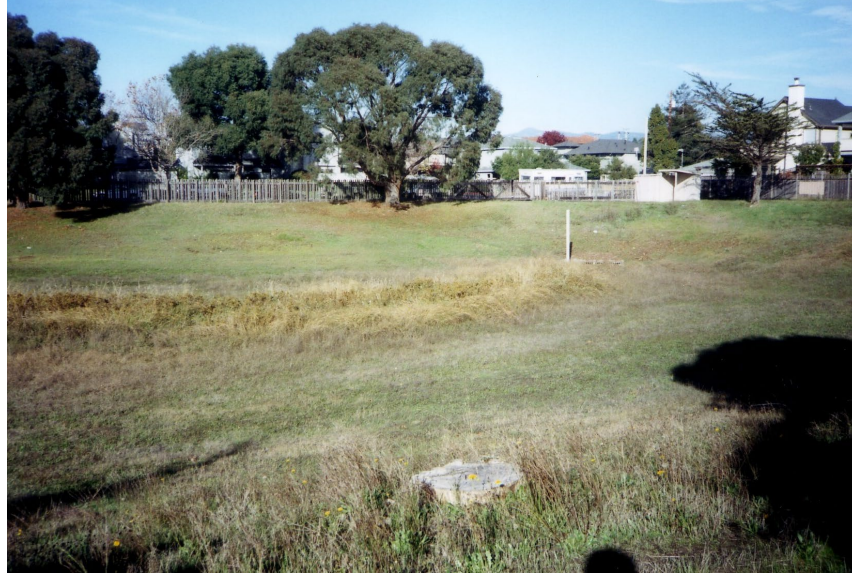
Figure 3.11. 38 th Avenue Stormwater Basin
