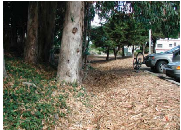
Existing Drainage Pattern at Base of Trees (Figure 49)
